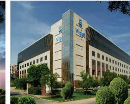
Vipul Plaza, Gurgaon
