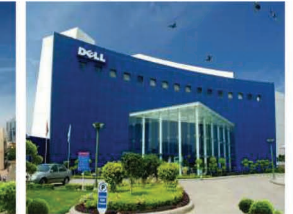
Vipul TechSquare, Gurgaon
